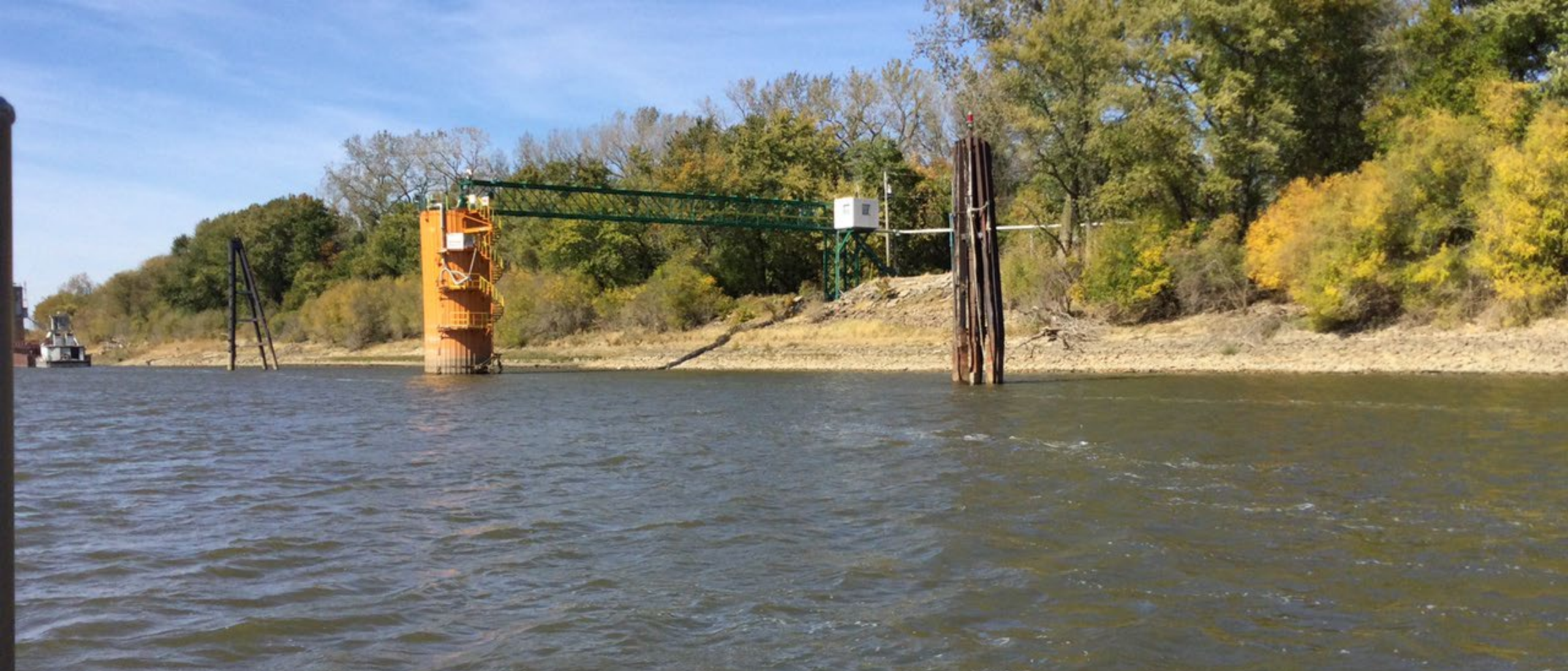
Anhydrous Ammonia Barge Loading (water side)
